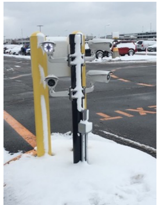
Heater Feature to prevent lens getting covered by snow.
